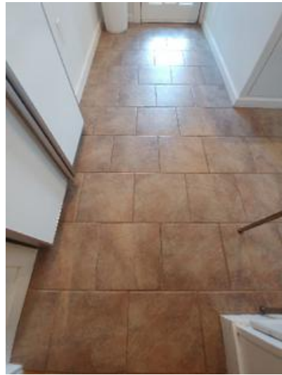
Flooring/Baseboard Taken on: 2018-10-03 12:11:14 Taken at: 32.7629140505, -79.9874196124 Image
