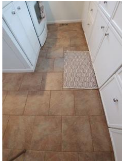
Flooring/Baseboard Taken on: 2018-10-03 12:11:30 Taken at: 32.762816045, -79.9875049149 Image
